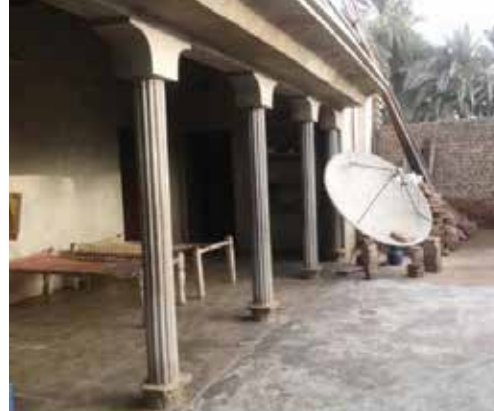
FIGURE 17: SATELLITE DISH INSIDE HOME
