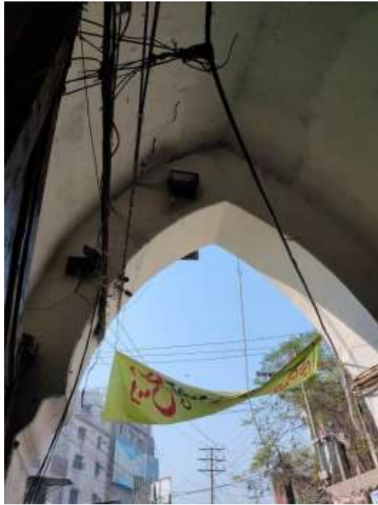
Electrical cables and light fixtures routed through and mounted on top of the gate structure, hung from metal grille and door.
