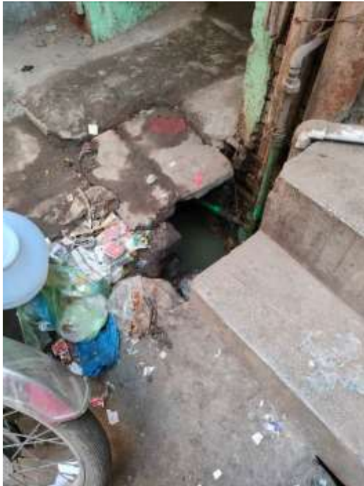
Open drains running along the facades on either side of the main bazaar. Such unhygienic conditions are a serious health hazard throughout the Walled City. The metal grate for the open drains is ineffective and fails to provide cover in certain sections.
