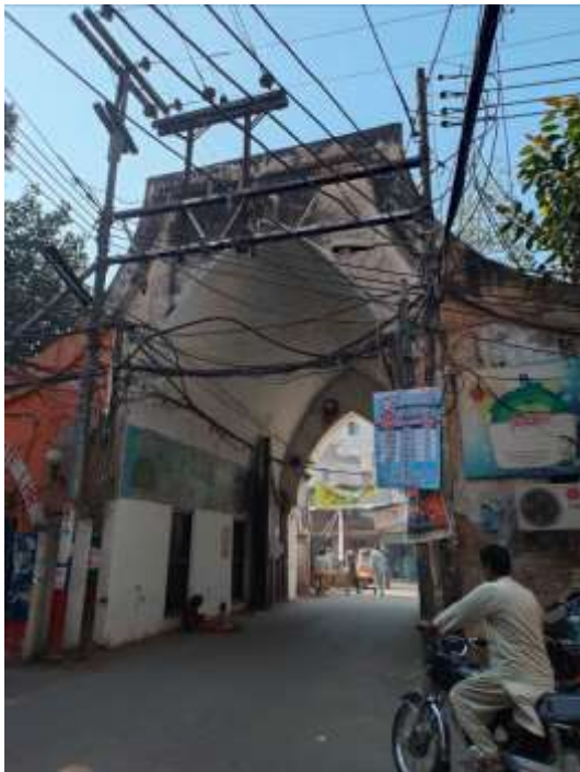
View of Bhatti Gate (front and back façade) showing web of electrical cables routed through the gate structure.
