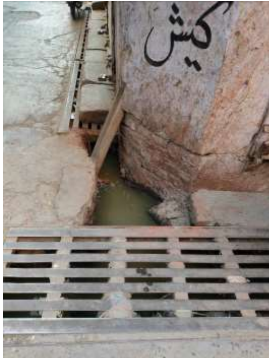
Open drains running along the facades on either side of the main bazaar. Such unhygienic conditions are a serious health hazard throughout the Walled City. The metal grate for the open drains is ineffective and fails to provide cover in certain sections.
