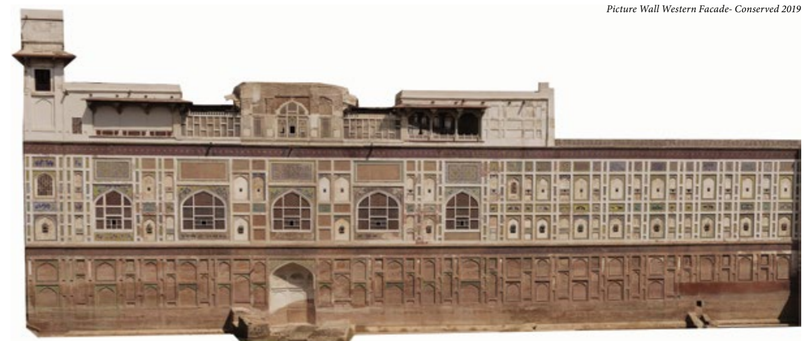
Picture Wall Western Facade- Conserved 2019
