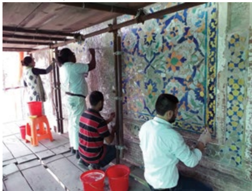
Conservators are consolidating Tile Mosaic Panel in prototype area Picture Wall- Source AKCSP
