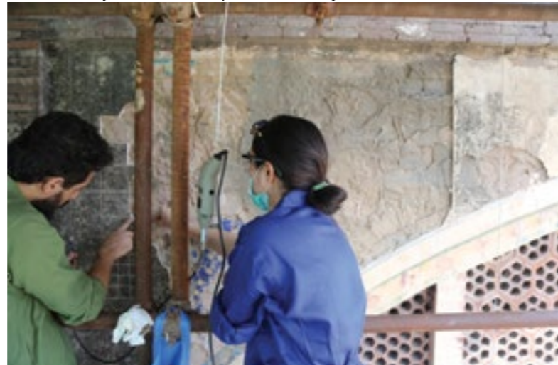
Removal of later layers of plaster from project area - Source AKCSP
