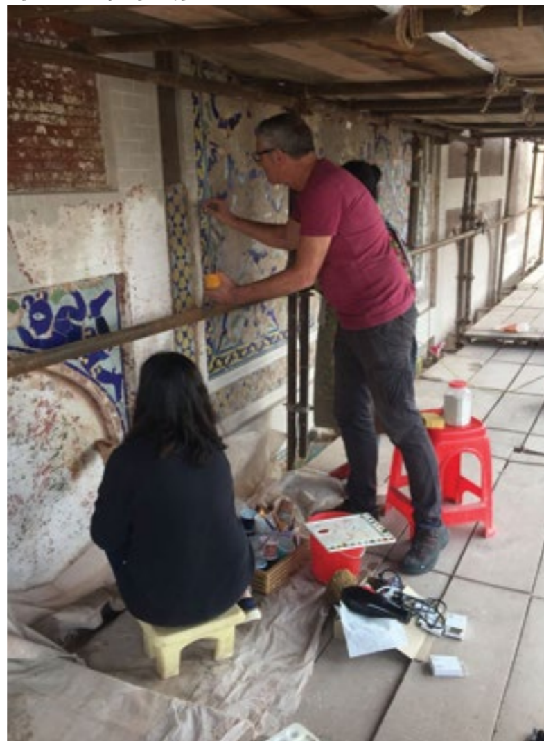
Consolidation of tile mosaic work by international experts - Source AKCSP
