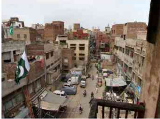
FIG. 29 REHABILITATION OF CHOWK MOTI TIBBA IN ZSV 5D. CLOCKWISE FROM TOP LEFT: EXISTING SITUATION; SECTION THROUGH PROPOSED REHABILITATED CHOWK; PLAN OF REHABILITATED CHOWK; PERSPECTIVE VIEW OF REHABILITATED CHOWK
