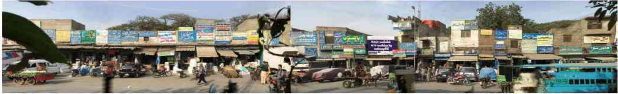
FIG. 49 ENCROACHMENTS CHARACTERISTIC OF THE EXISTING SITUATION ON CIRCULAR ROAD BETWEEN SHAH ALAMI AND MOCHI GATE
