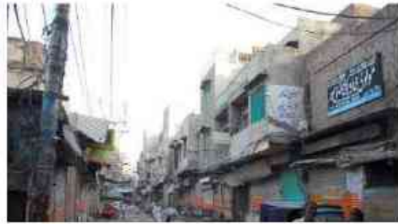
VIEW OF THE DELHI GATE BAZAAR FROM THE DELHI GATE BEFORE (TOP) AND AFTER (BOTTOM) REHABILITATION WORK WAS CARRIED OUT
