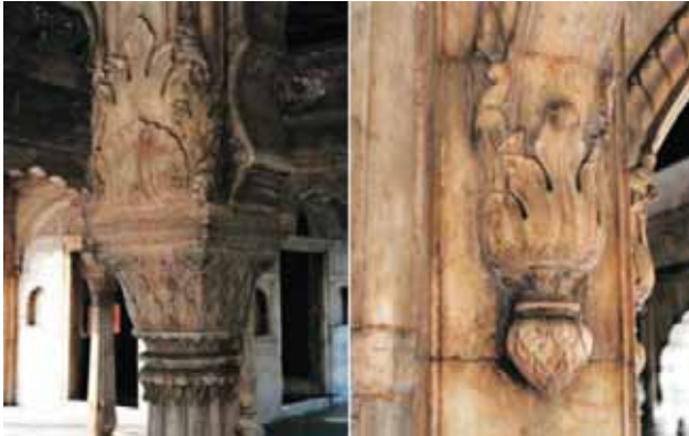
Figure 19: Detail of Impost and Springer in Marble Carving Related to Jehangir's Period.
