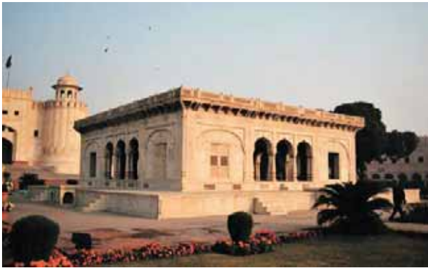
Figure 7: A View of barhdari from North-West Side
