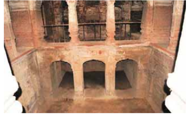
Figure 14: View of Basement and Sub-Basement
