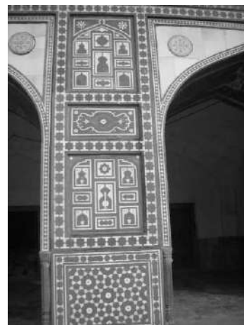
Figure 12: Panels of stone inlay after conservation
