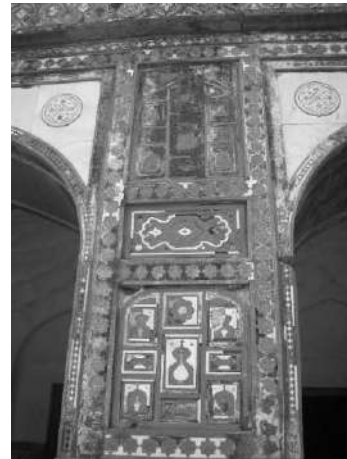
Figure 11: Panels of stone inlay before conservation
