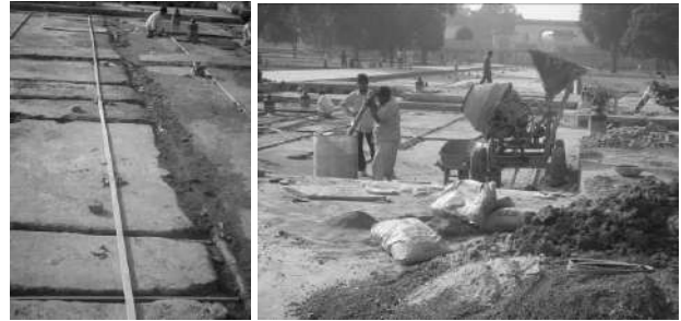
Figures 5 & 6: The laying out of G.I pipes in Shalamar garden
