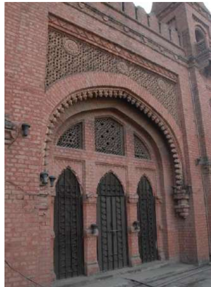
Figure 9 Upper Storey of Vestibule
