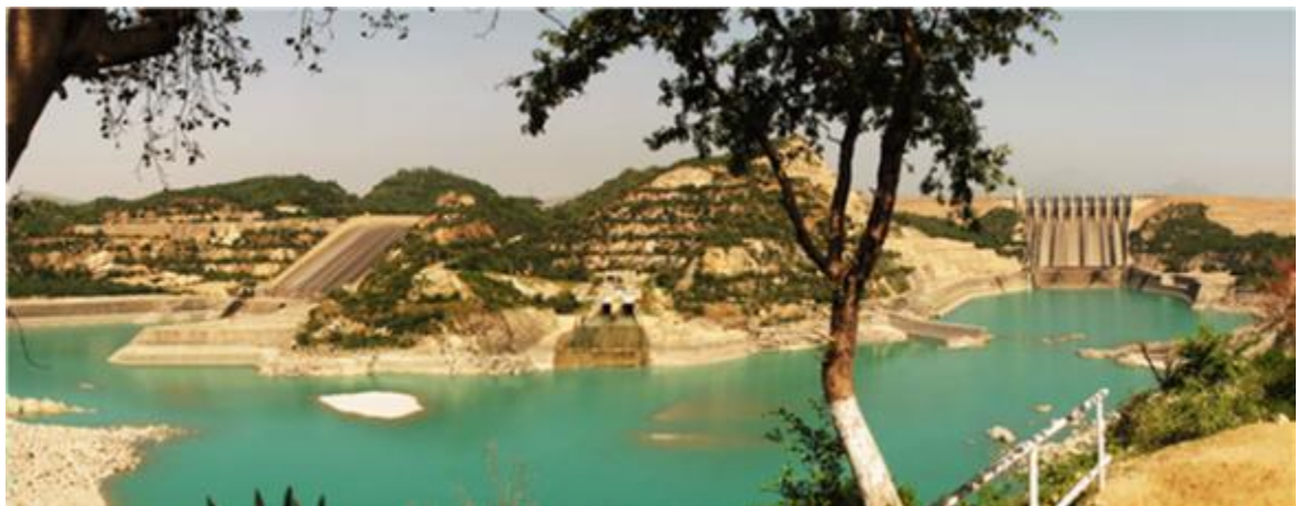
Figure 3-2: View from downstream looking at T5 outlet between the service and auxiliary spillways
