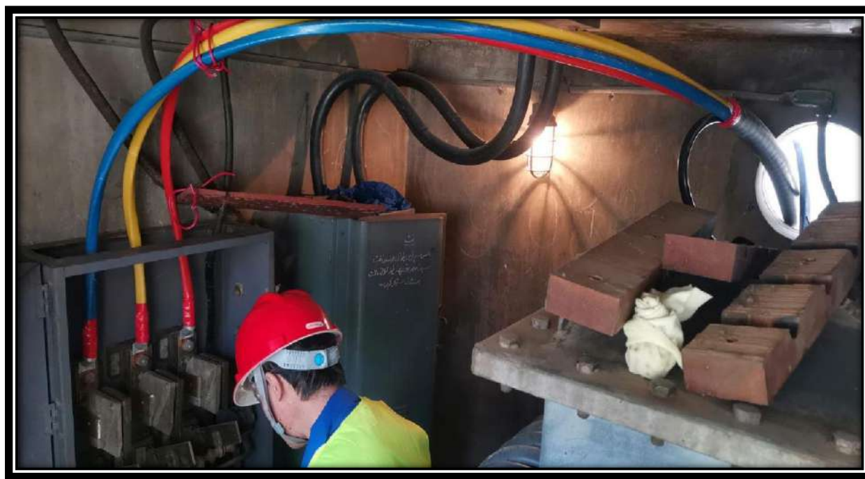
Connection of Temporary Power Supply to Emergency Panel in Switchyard
