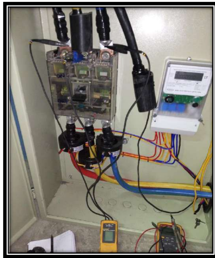
Megger Testing of Newly Installed Cable
