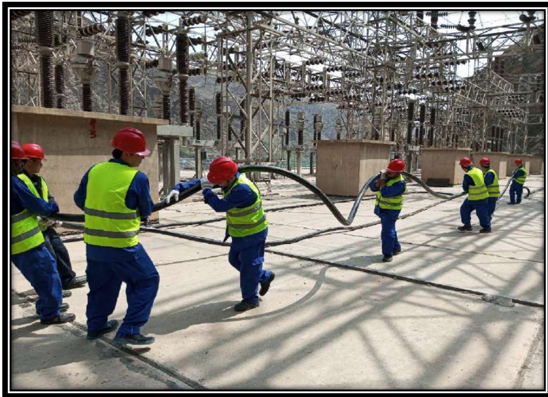
Cable Laying Started in Switchyard
