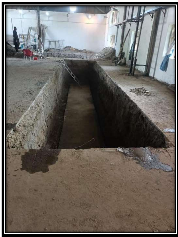
Foundation works are in progress for Heavy duty horizontal Lathe Machine
