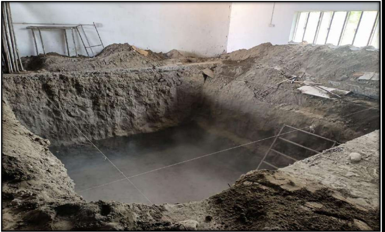
Foundation works for Vertical lathe Machine are in progress
