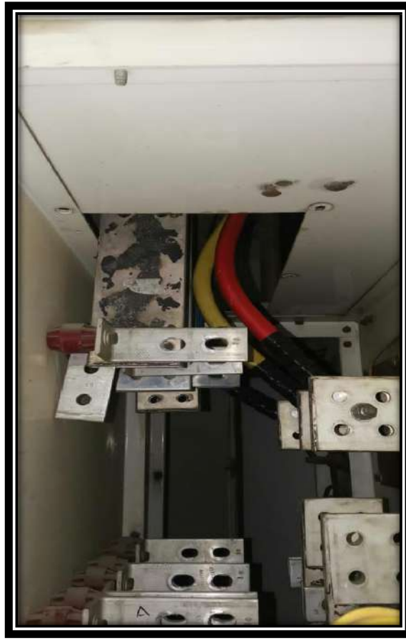
Connection of Temporary Power Supply to Excitation Panel of Unit 6
